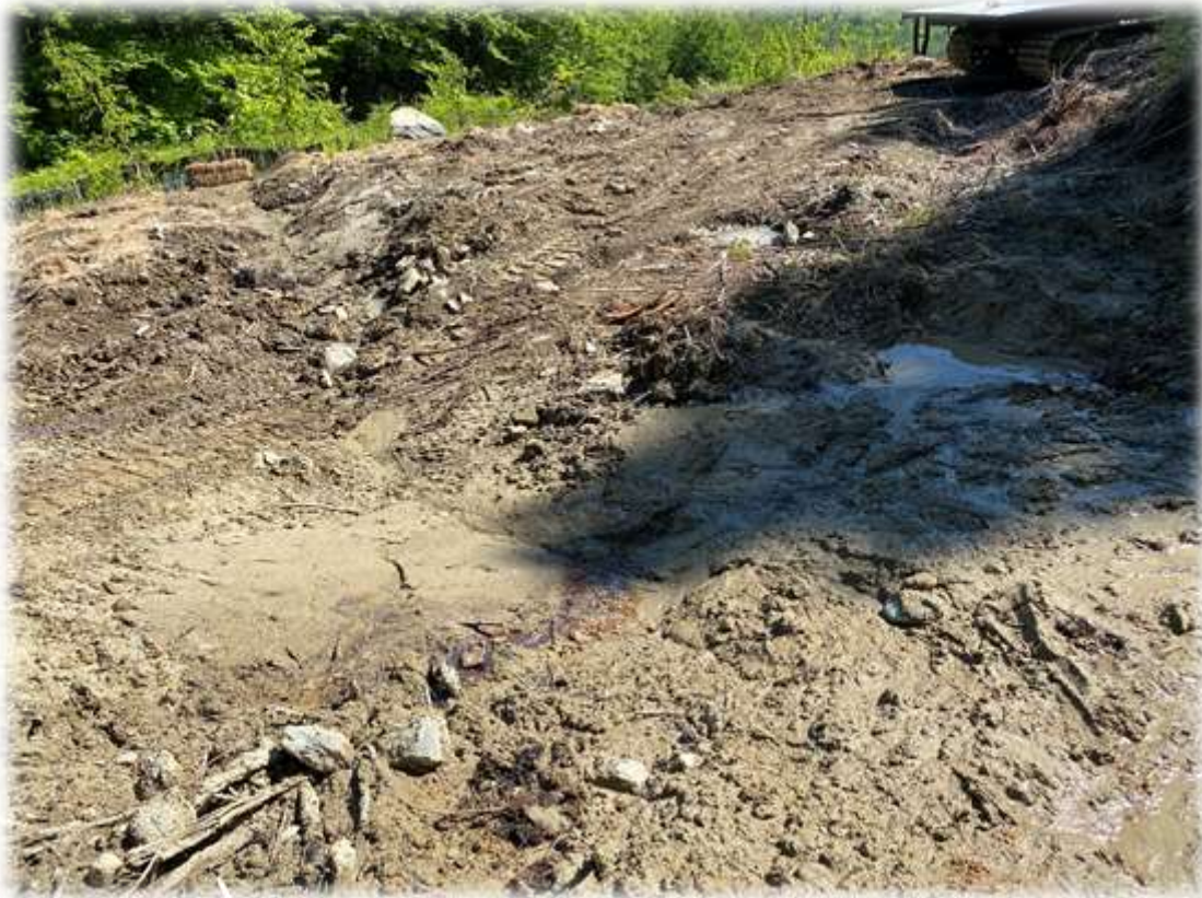
Photo #6: Water bars have captured groundwater flows passing through the access road area.
