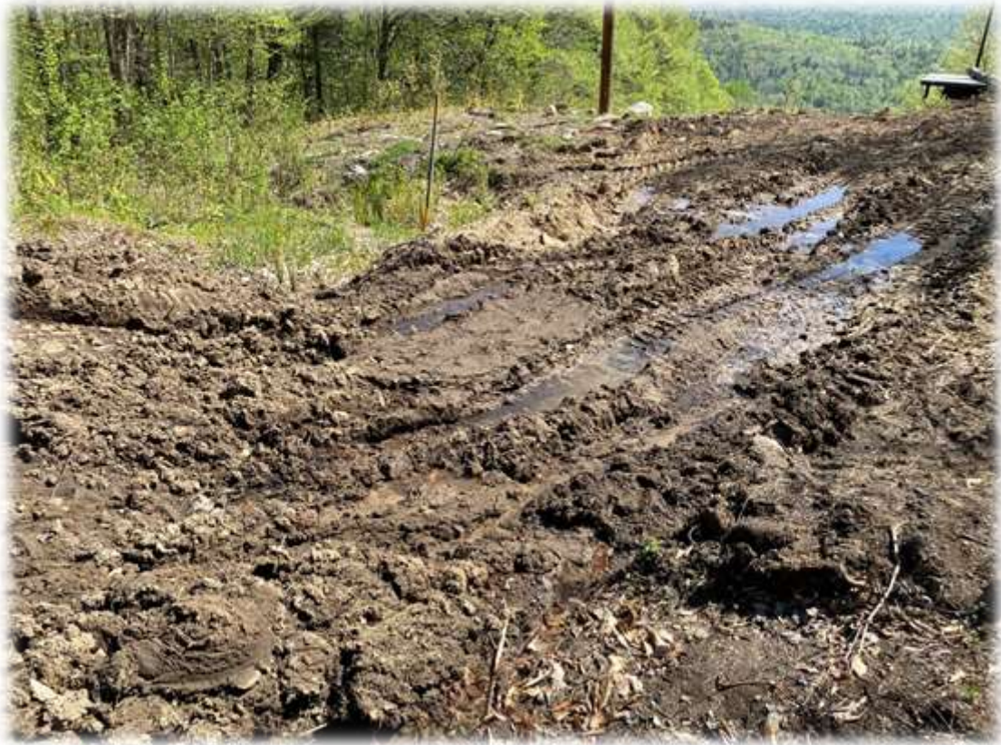
Photo #7: Another view of the same stream crossing.
