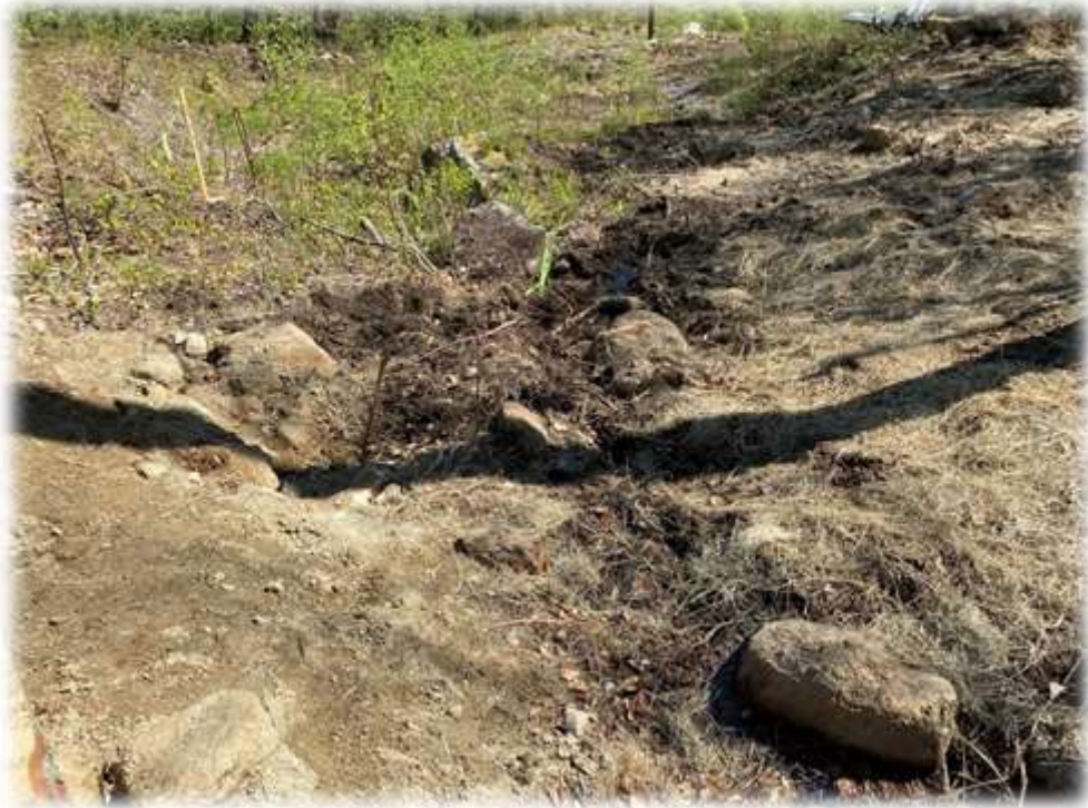
Photo #9: It appears this location adjacent to structure 28 may have been a stream crossing that has been disturbed (not matted).
