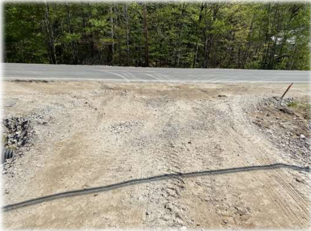
Photo #1: Roxbury Road pavement is clear of soil debris at the intersection with the SCADA building driveway.
