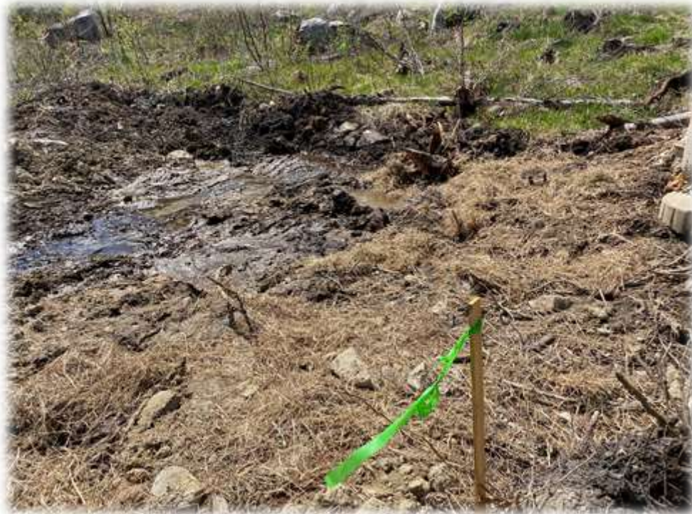
Photo #10: The two green flagged stakes are 15' offset stakes meaning the structure would have been located in the center of the flowing water of the drainage swale (near the rocks).
