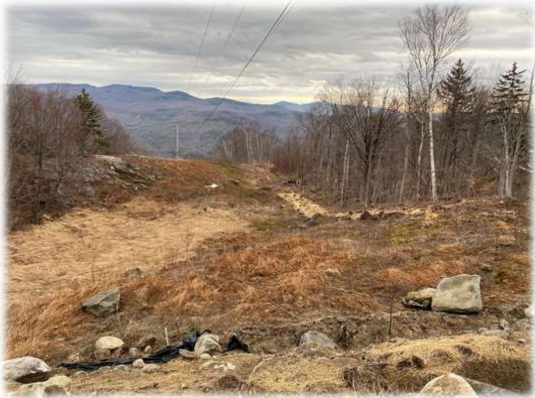
Photo #1: Cut/cleared areas along the existing transmission line have been completed to the top of the mountain (tower 1 location).
