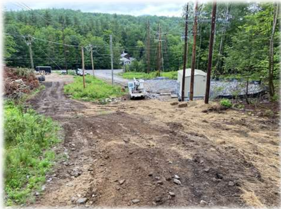
Photo # 8: The SCADA Building and driveway area remain secure and stabilized.
