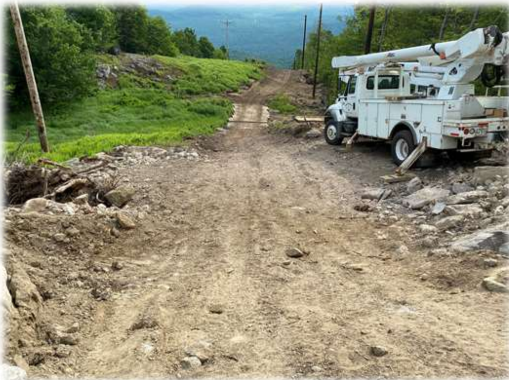
Photo #2: The corridor remains dry, mats have been placed in wetland areas, and disturbed areas mulched.
