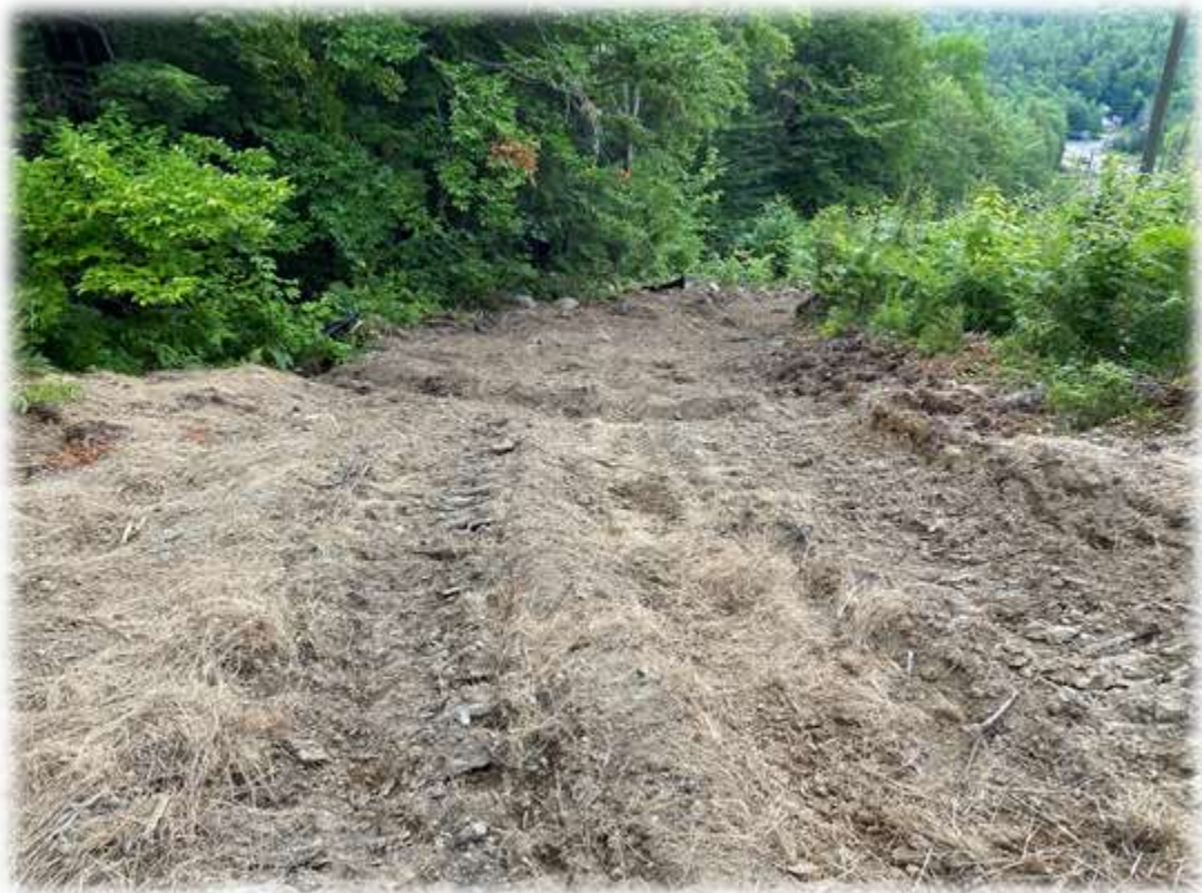
Photo #6: Water bars have been reconstructed and have adequate stabilized outlets.
