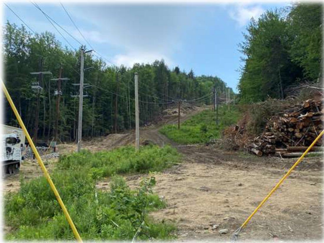
Photo #11: an overview of the lower end of the corridor.
