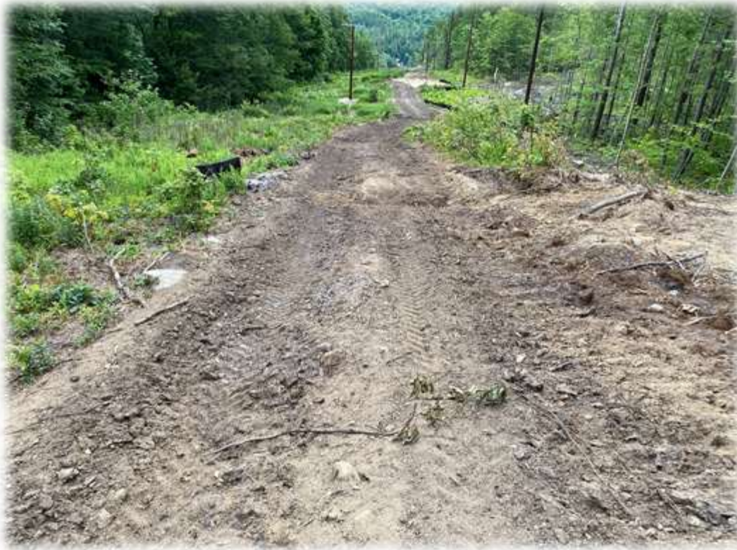
Photo #3: Water bars have been created along the corridor access road. The bars flow to a stabilized area with silt fence barrier to collect potential sediment wash
