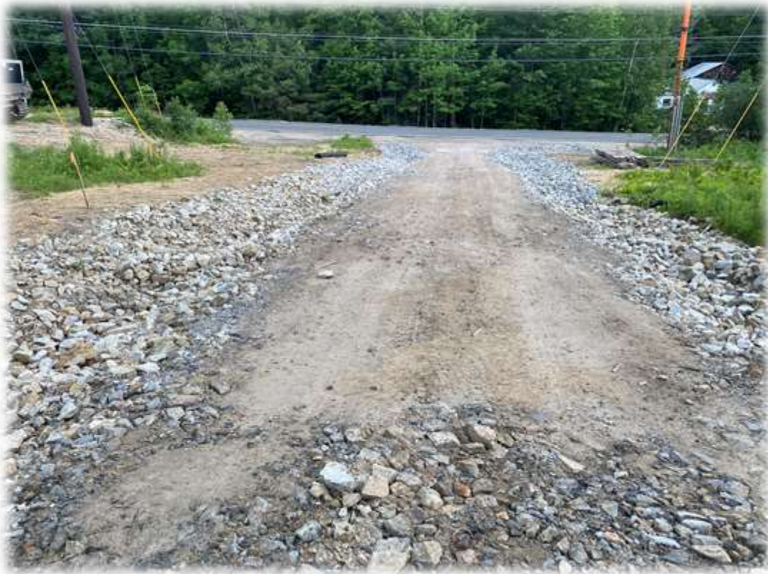
Photo 9: The SCADA driveway has been completed.
