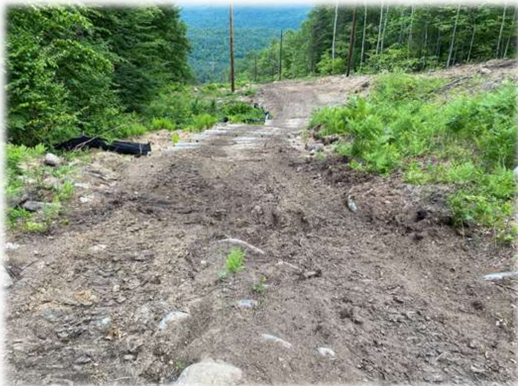
Photo #2: Water bars have been created along the corridor access road. The bars flow to a stabilized area with silt fence barrier to collect potential sediment wash.
