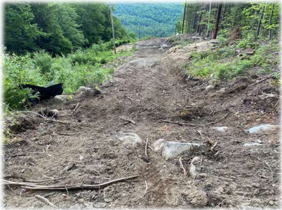
Photo #5: Water bars have been reconstructed and have adequate stabilized outlets.
