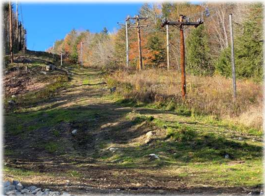
Photo #10: The lower end of the transmission corridor has some vegetative growth. More growth is needed in bare areas. A heavy application of hay mulch is needed in bare soil areas.
