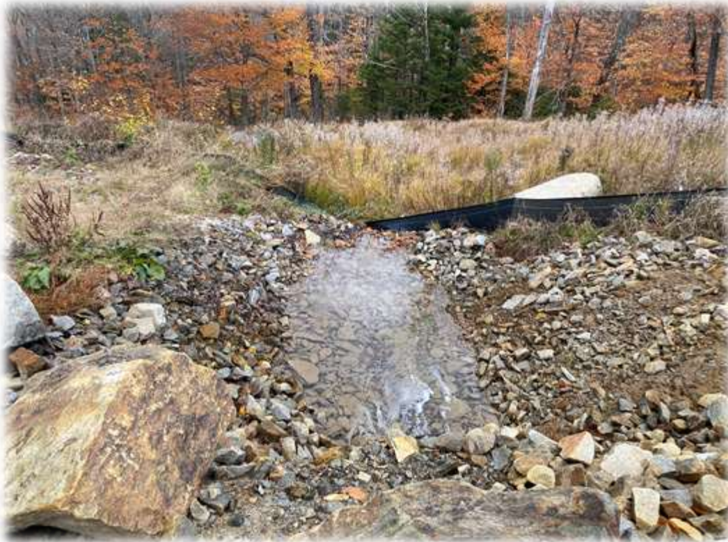
Photo #3: Stream beds do not seem to be passing significant sediment. The plunge pool outlet has been cleared of sandy debris.
