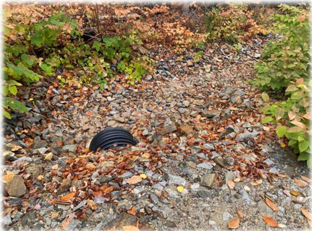
Photo #2: Sediment within the rocky plunge pool area across from the driveway entrance has been removed. No new sediment buildup noted.
