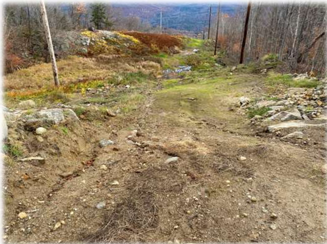
Photo #4: The upper portion of the transmission corridor access road coming into the RoxWind Towers portion of the project has been restored. Water bars have captured and diverted upland areas into stabilized areas. A significant catch of vegetation is becoming established. Some erosion is beginning to occur that should be redirected at the rock barrier along the road.
