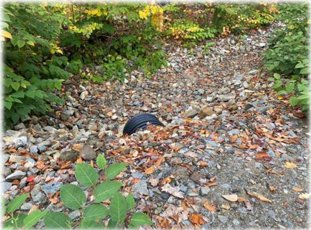
Photo #2: Sediment within the rock-plunge pool area across from the driveway entrance has been removed.
