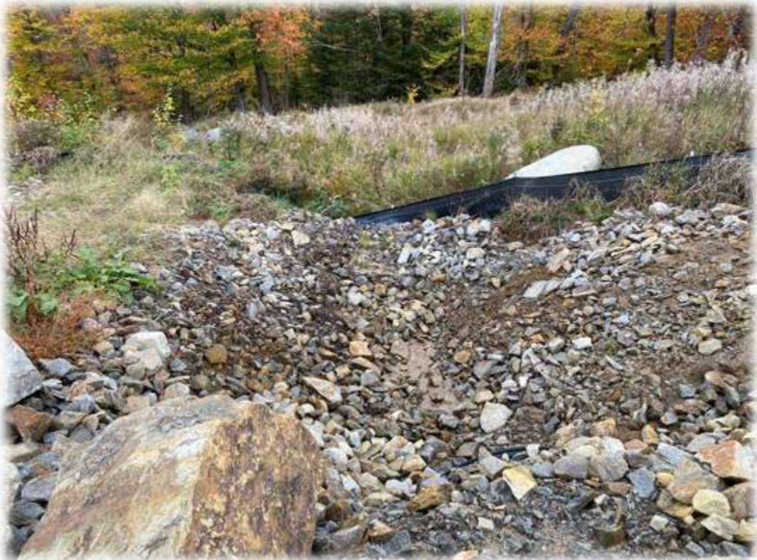
Photo #4: Stream beds do not seem to be passing significant sediment. The plunge pool outlet has been cleared of sandy debris.
