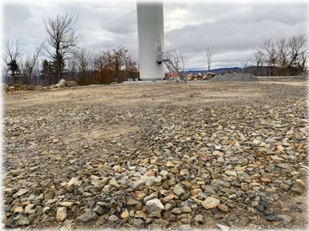
Photo #7: No activities are ongoing at Tower 2 location.
