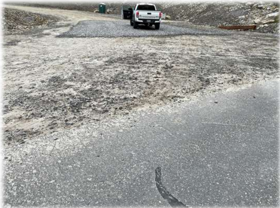
Photo #2: The stabilized construction entrance has new stone installed.
