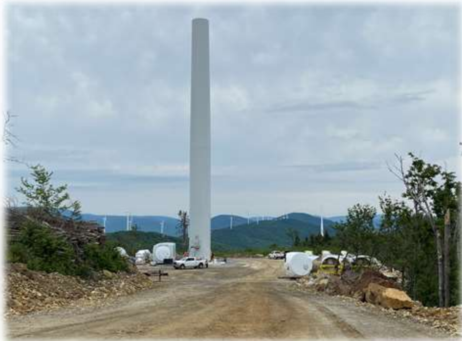
Photo #9: The base and mid-section of Tower 3 has been set. No significant changes since last week.
