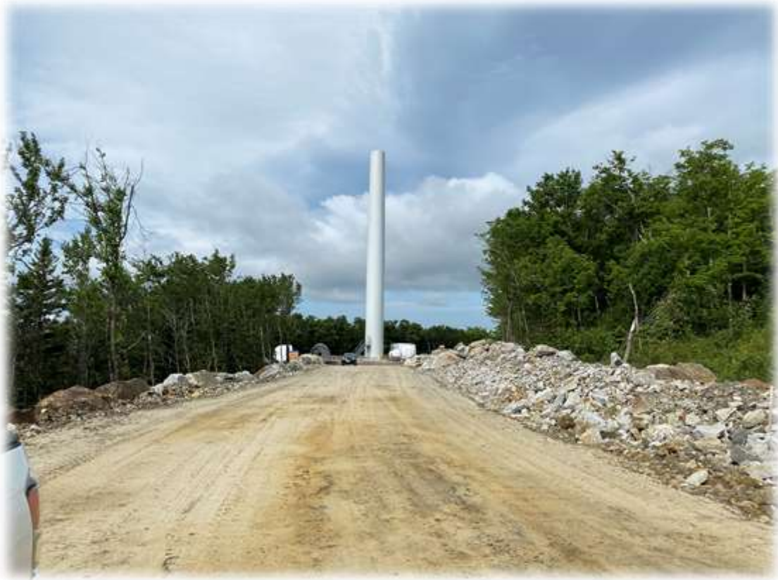
Photo #7: The base and mid-section of Tower 4 has been set.
