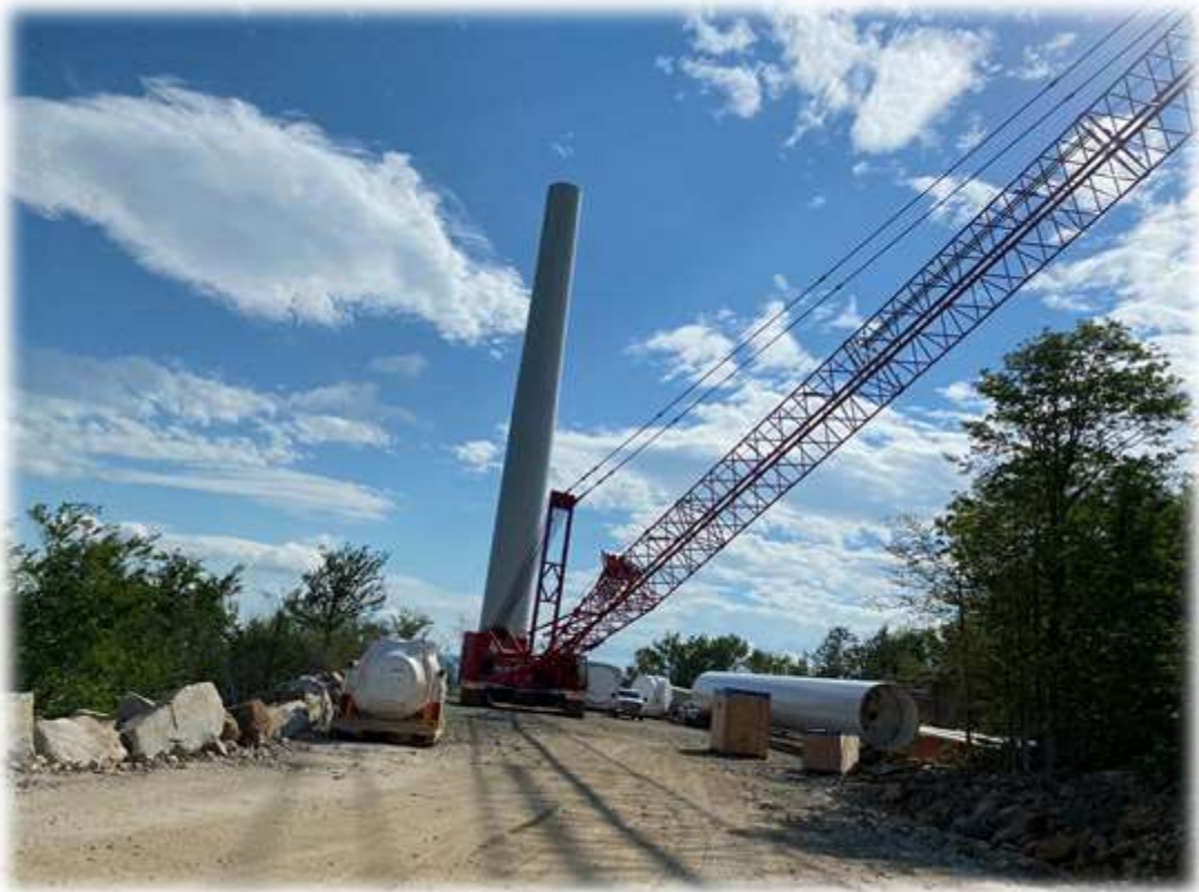
Photo #5: The base and mid-section of Tower 2 has been set.
