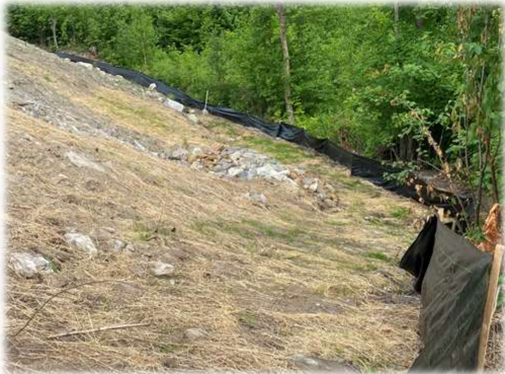
Photo #8: Grass is beginning to establish itself along the 180 degree corner near Tower 1.
