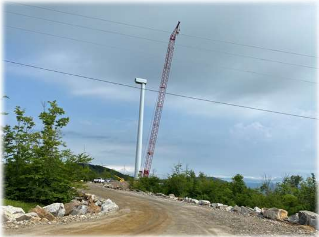
Photo #4: Tower 1 has been set including the Nacelle at the top of the tower.
