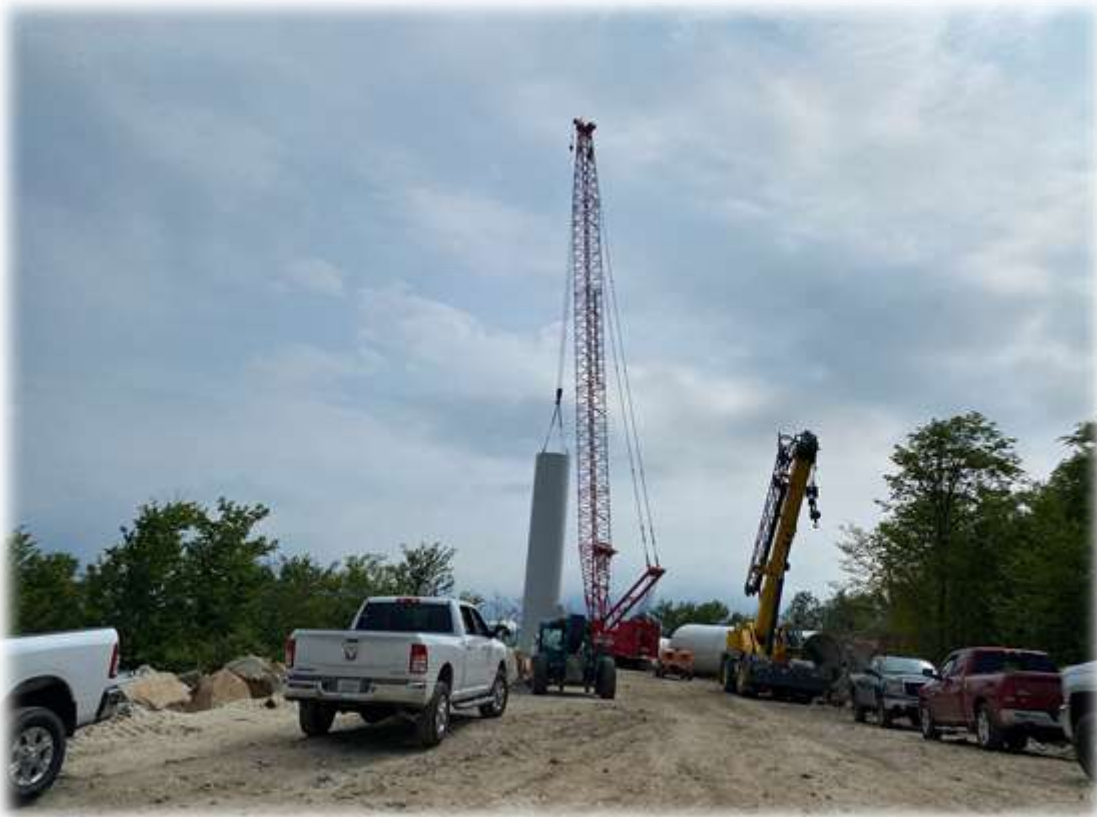
Photo #5: The base section of Tower 2 is being set.
