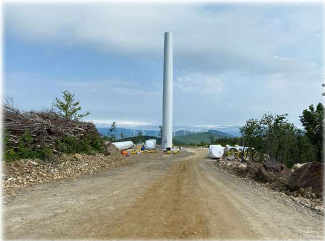
Photo #6: The base and mid-section of Tower 3 has been set.
