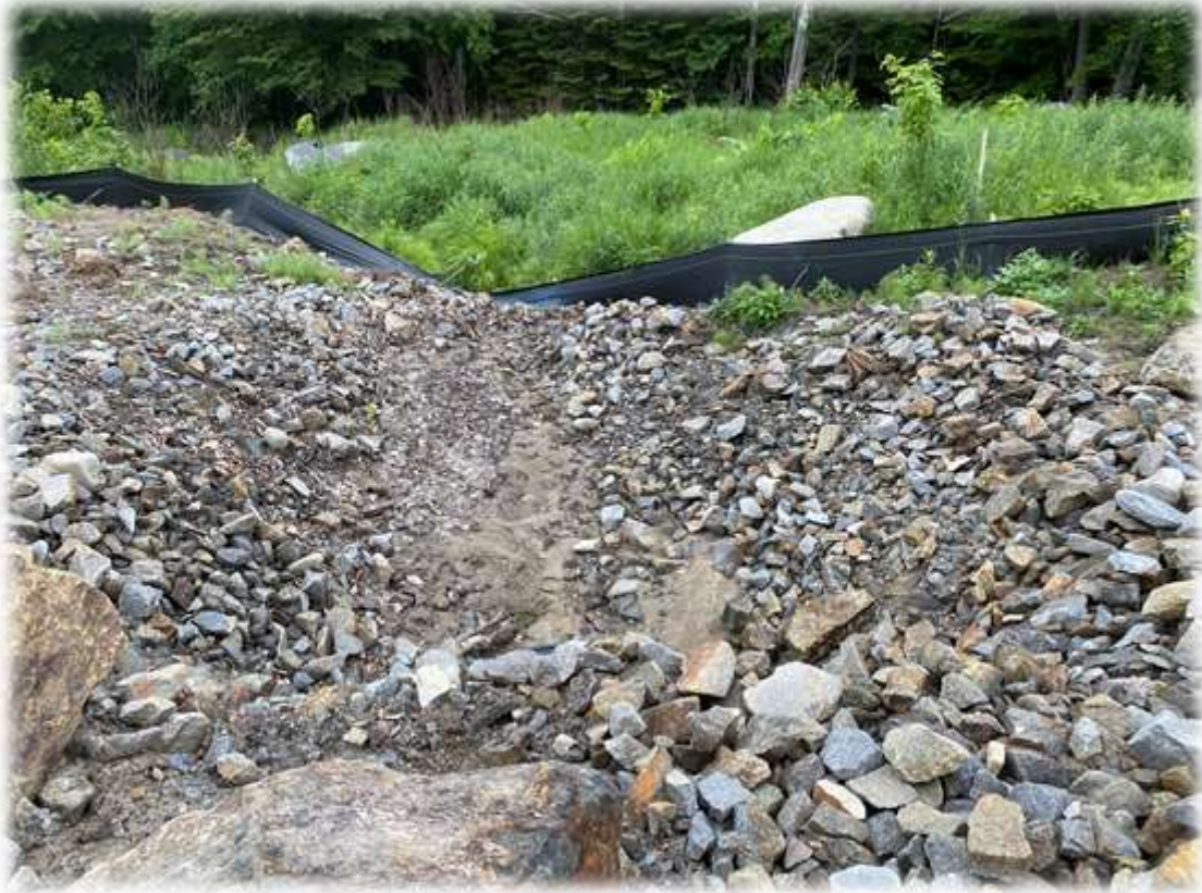
Photo #3: Even with a little rain last night, many of the streams/drainage swales have no, or little, water flowing.
