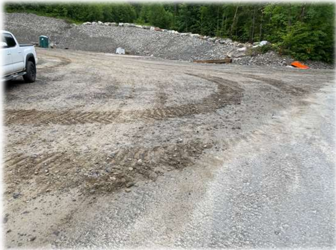
Photo #2: The stabilized construction entrance been removed in order to bring tower sections and blades into the project.
