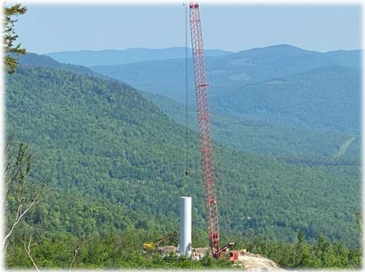
Photo #5: The base section of Tower 1 is being installed.
