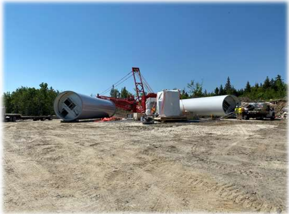
Photo #4: Sections of Tower 3 have been delivered to the site.
