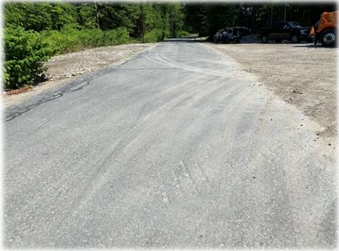
Photo #1: Horseshoe Valley Road is clear of soil debris from the project.
