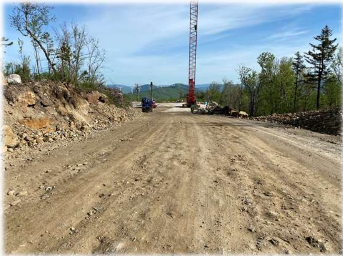
Photo #6: A large crane has been assembled at Tower 3.
