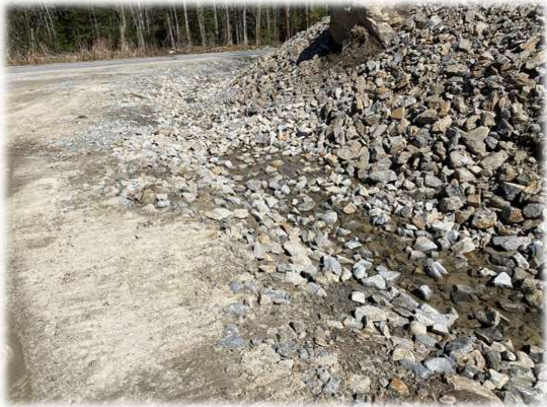
Photo #3: Water within the ditch is clear. Sargent has cleaned the ditches of sediment (winter sand accumulation) from the top of knoll to Horseshoe Valley road as a first work priority.
