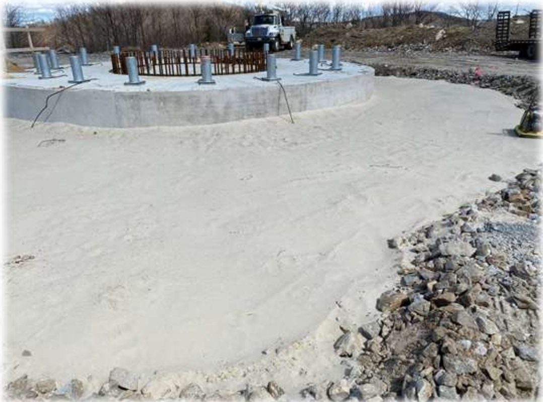
Photo #6: Tower 1 base have been backfilled and grounding system installed.
