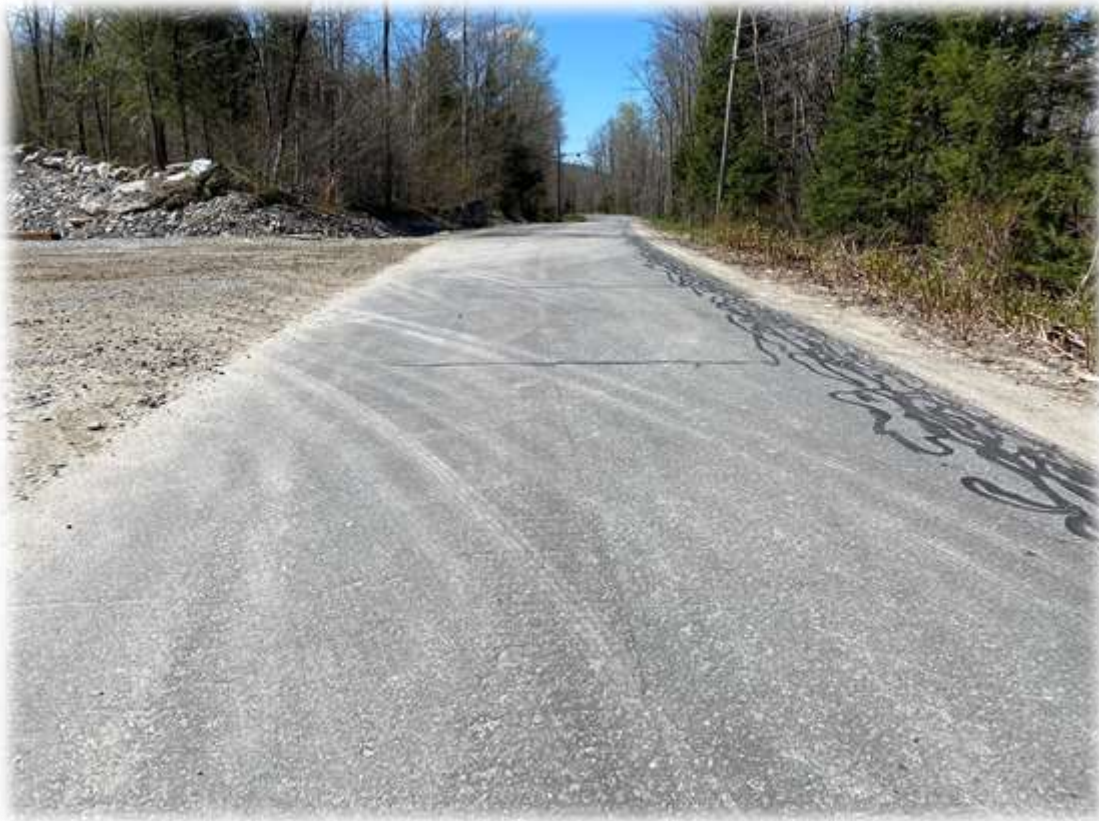
Photo #1: Horseshoe Valley Road is clear of soil debris from the project. The stabilized construction entrance still has some life left to the crushed rock entrance.
