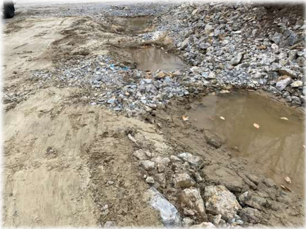
Photo #3: Water within the ditch is clear. Sargent is to clean the ditches of sediment (winter sand accumulation) from the top of knoll to Horseshoe Valley road as a first work priority.
