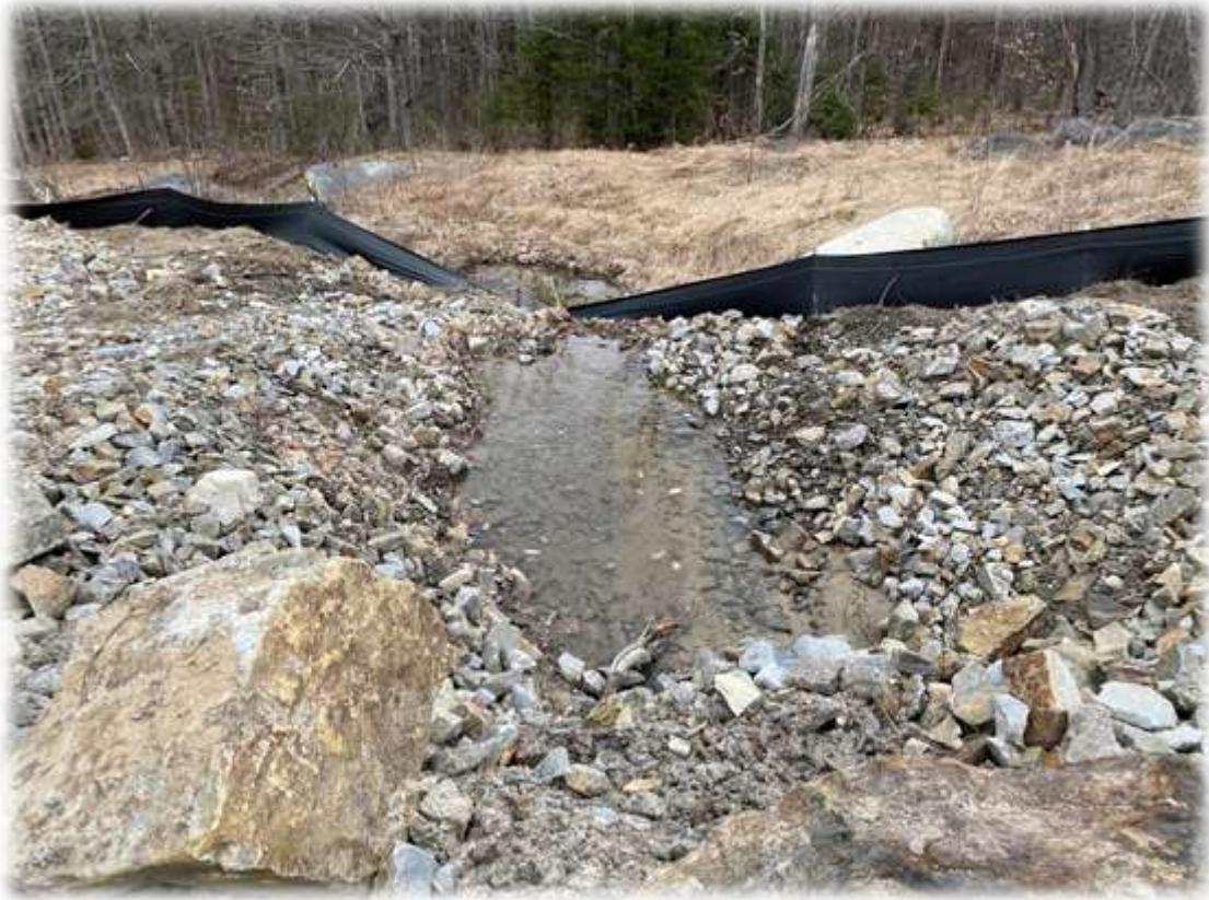
Photo #5: In general, all culverts are discharging clear water.
